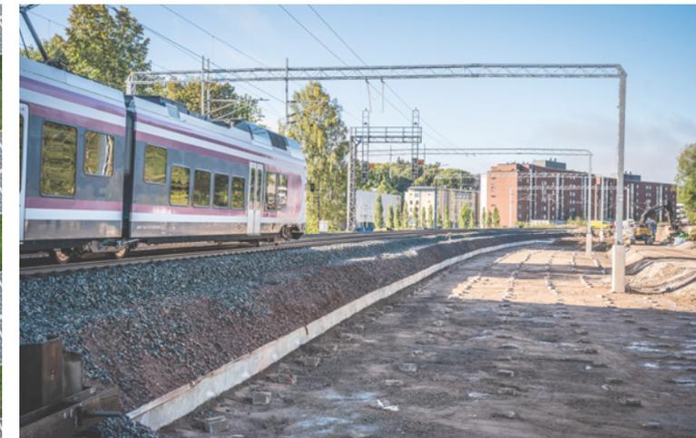
**We started work on the Espoo Rail Line area contract 3, which is located between Koivuhovi and Espoon keskus.** In the summer of 2024, during a five-week track possession, we carried out a total of approximately 70,000 m<sup>3</sup> of soil cutting and replacement of materials, approximately 17,000 metres of piling, 35,000 m<sup>3</sup> of excavation, 375,000 kg of reinforcement and 4,500 m<sup>3</sup> of concreting in the contract area.
