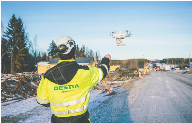
**We deployed two autonomous drones in the national road 6 at Korja project in Kouvola, marking the first time autonomous drones were used at a construction site in Finland.** Drones substantially increase the opportunities for using artificial intelligence at infrastructure sites. Independent systems that include drones can be located virtually anywhere and are not tied to the location of a situation room, for example.
